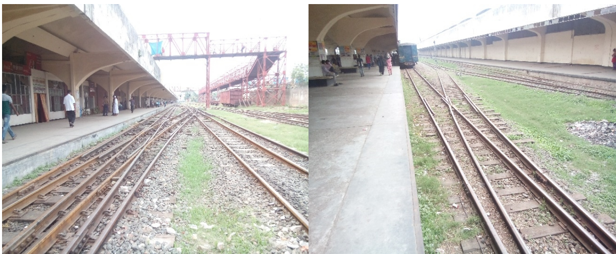
Figure 2. A DG (one the left) & a SG (one the right) Points and Crossing at Kamalapur Railway Station
