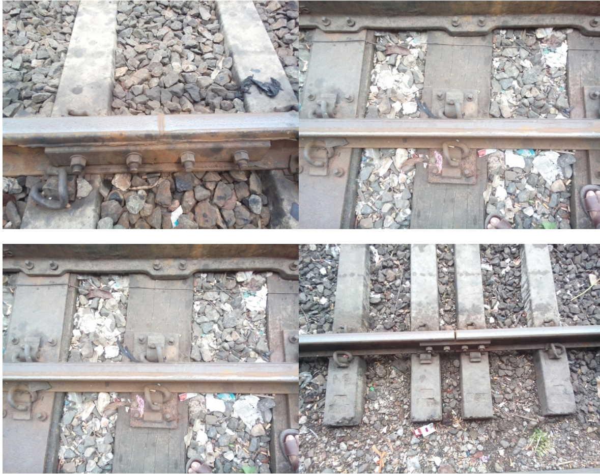
Figure 2. Rail joints and fasteners near Kamalapur Railway Station.
