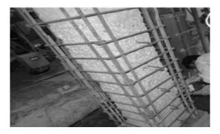
Figure 1. Additional Reinforcement Provided for Strengthening.
