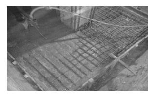
Figure 4. Pouring of Micro Concrete.
