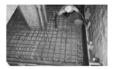
Figure 2. Application of Epoxy Bonding Agent.
