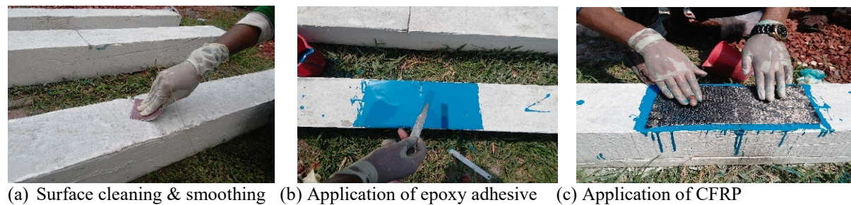
Figure 3. Surface cleaning, smoothing and application of epoxy adhesive & CFRP to the selected area
