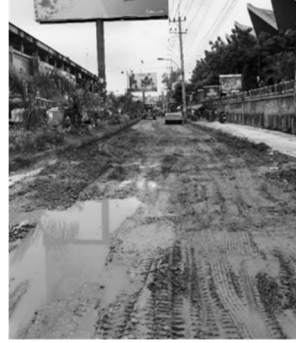
Figure 4. On street construction
