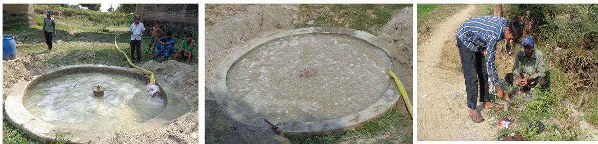
Figure 5. Measuring recharge capacity of recharge well and taking water level record
