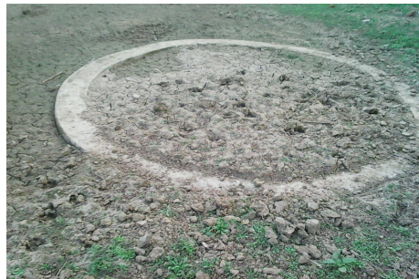
Figure 6. Clogged Recharge well at Paramanondopur
